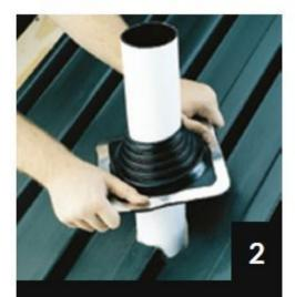
Slide the Master Flash® down the pipe, using a non-petroleum-based lubricant to ease installation.
