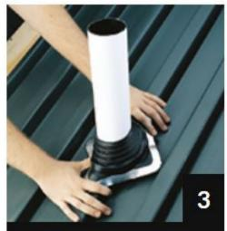
Press Master Flash® down, bending it to conform to roof profile or roof irregularities. A blunt tool will help to form flashing to tight roof angles.
