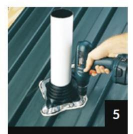
Use fasteners to complete sealing. For a secure installation, fastener spacing must not exceed 1.5" (38 mm).
