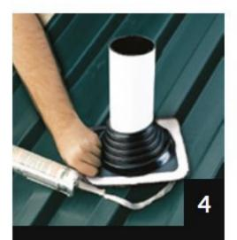
Apply sealant between the base of the flashing and the roof.
